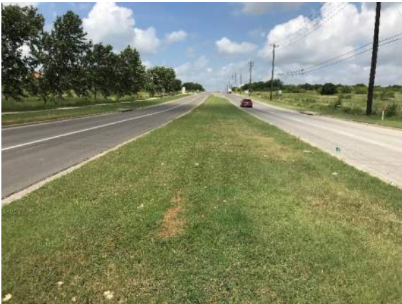
Photo 3. Kohlers west of the UPRR crossing. The photo is facing west.
