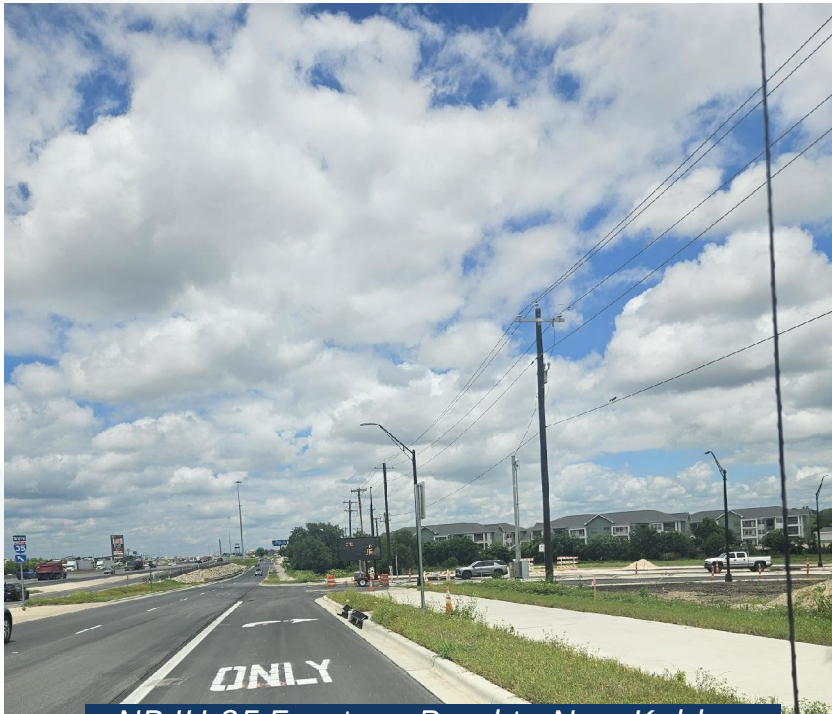
NB IH-35 Frontage Road to New Kohlers to Seton Intersection
